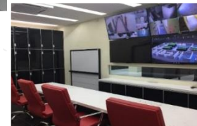
DCIM ( Data Center Infrastructure Monitoring
