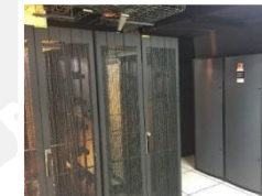
Computer Room Air Conditioning System
